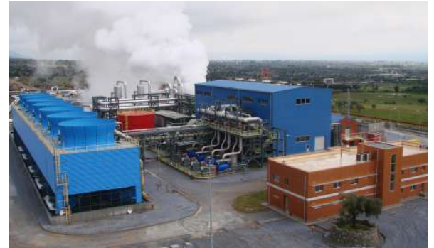
Germencik - 45MW - Germencik, Turkey. The largest geothermal power plant in Turkey comprises eight wells with drilling depths between 1,000 and 2,400 meters.
